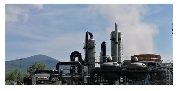
Residues: adsorbent and filtering materials are employed in AMIS to trap mercury and hydrogen sulphide from gas
